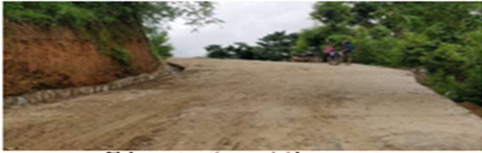
Slab construction as rigid pavement
