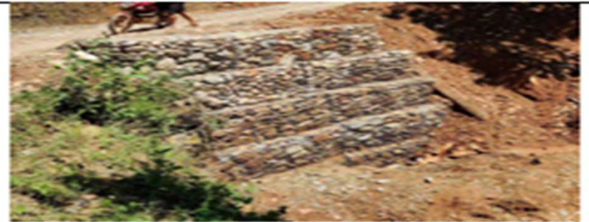
Gabion wall construction
