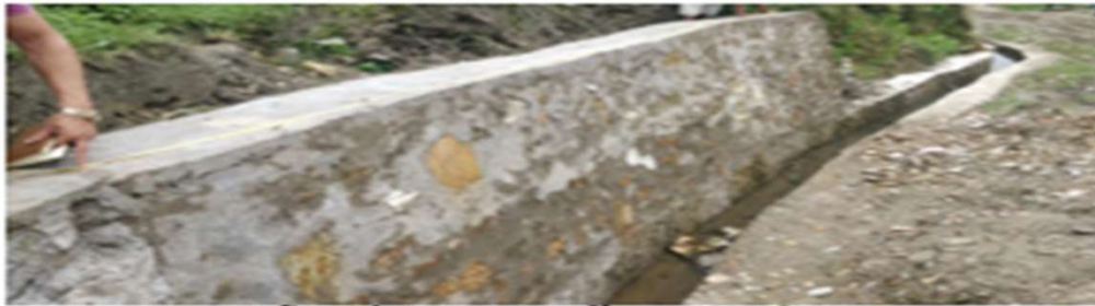
Some masonry wall construction
