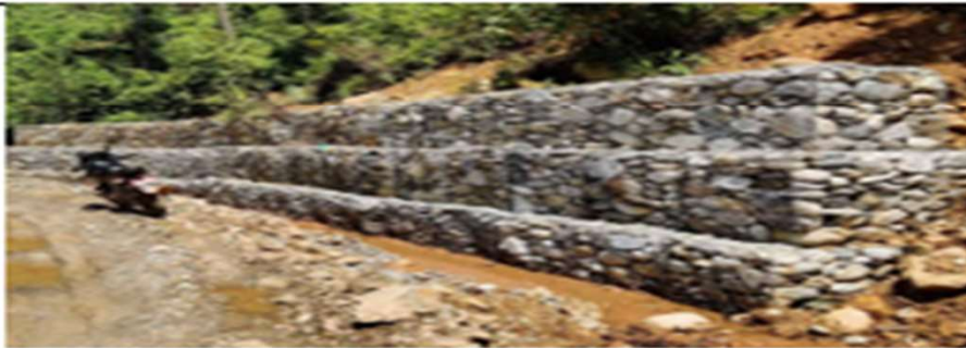
Gabion wall construction
