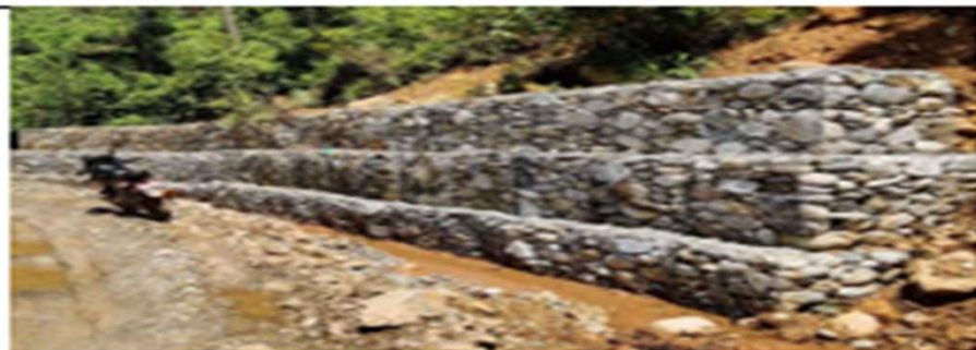
Gabion wall construction
