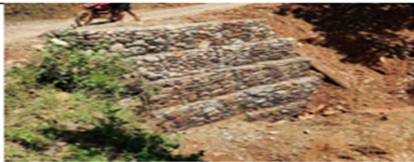
Gabion wall construction
