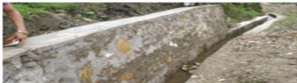
Some masonry wall construction
