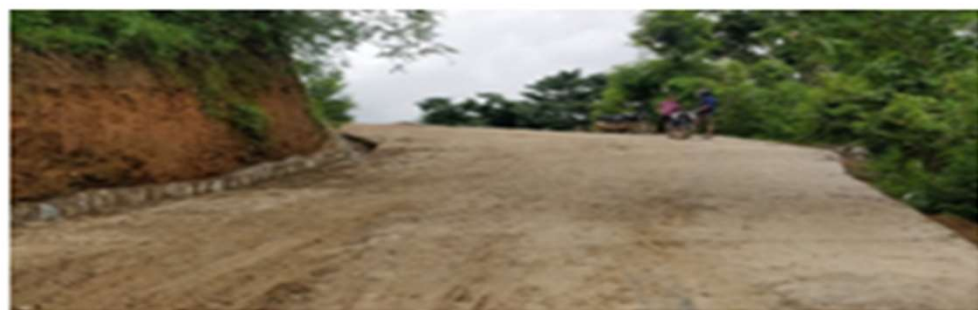
Slab construction as rigid pavement
